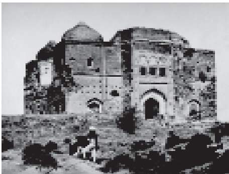
Fig. 11.8 A mosque on the Delhi Ridge, photograph by Felice Beato, 1857-58 After 1857, British photographers recorded innumerable images of desolation and ruin.
