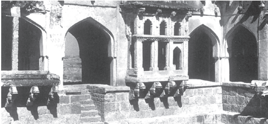
Fig. 7.32 Part of a structure known as the queen's bath
